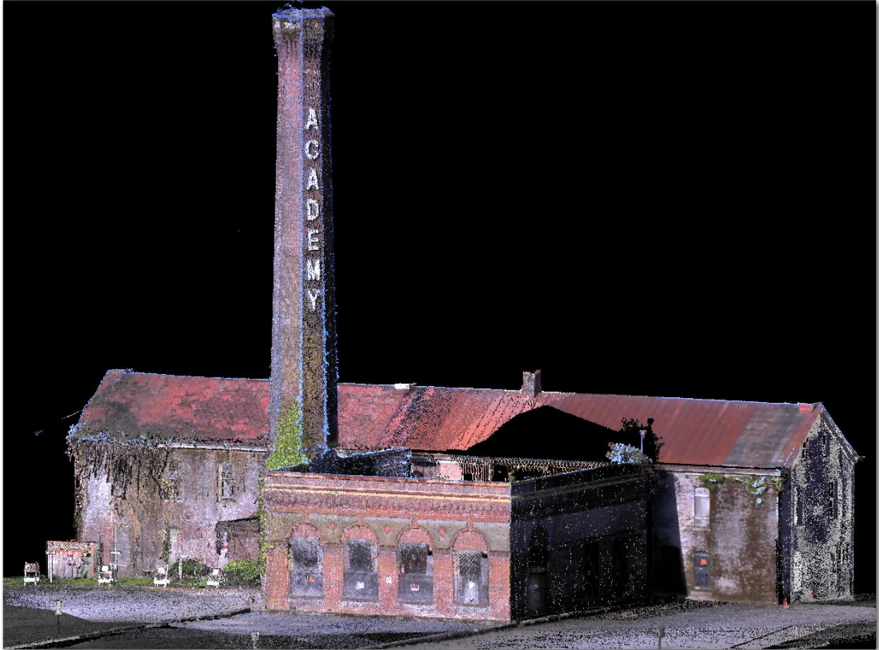
Laser scan of Boiler Plant (foreground) and Laundry Building (background), April 28, 2019, Olson Engineering
