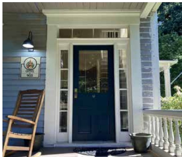
SIDING REPAIRS FOR A BUILDING ON OFFICERS ROW
