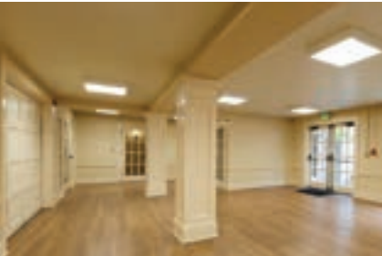
RED CROSS BUILDING, LOWER LEVEL
