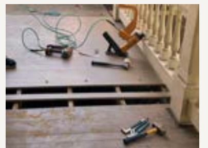
PORCH REPAIRS - SUMMER 2025
