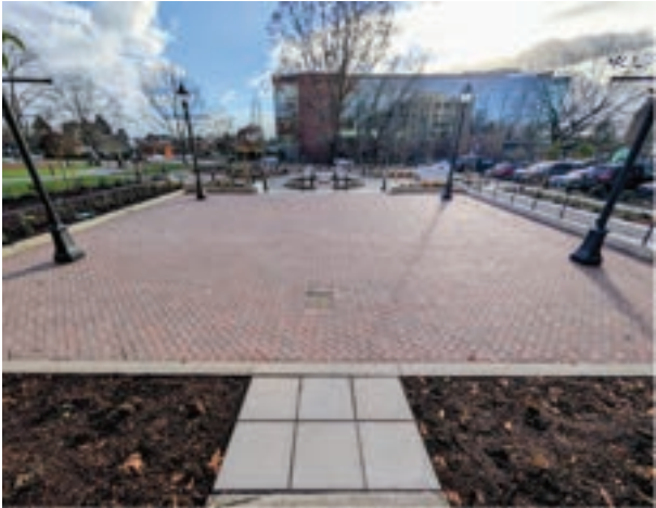
COMPLETED PLAZA IN NOVEMBER
